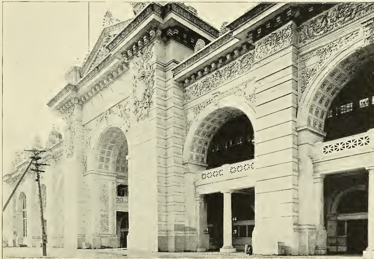
MAIN ENTRANCE OF THE MINING BUILDING, Facing Wooded Island.
